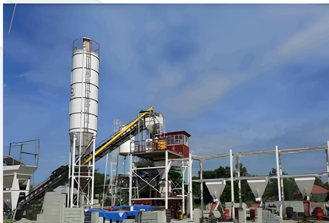
SUPPLY BATCHING PLANT ( BULACAN )
